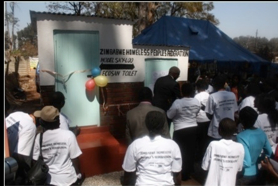
Eco-san toilet block, Harare
