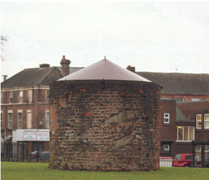
Figure 9: Ventilation shaft for the Victoria tunnel, Helena Street.
