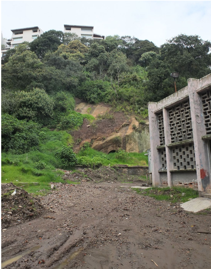
Figure 16.2. Collapsed hillside at a SACMEX facility
