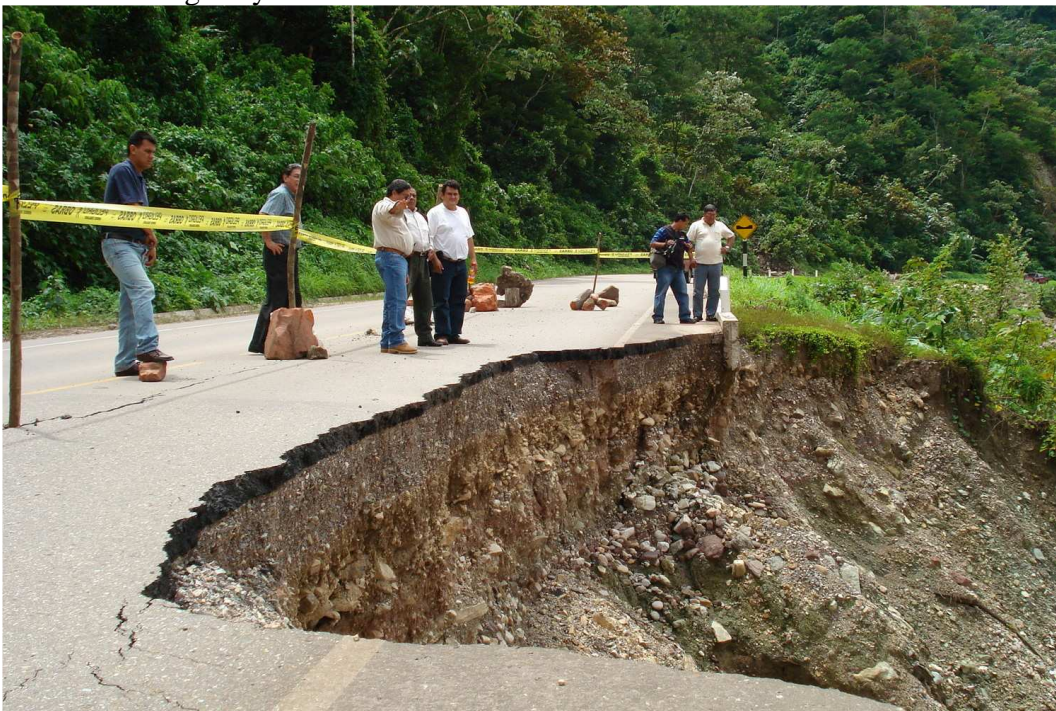
Road failure along a section of the soon-to-be concessioned Central Amazon Highway, part of IIRSA. Photo courtesy of the Ucayali Chamber of Commerce, Tourism and Industry. February 10, 2007
