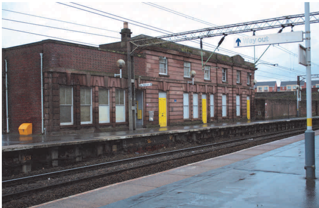
Figure 12: Edge Hill station (1836), south side buildings.
