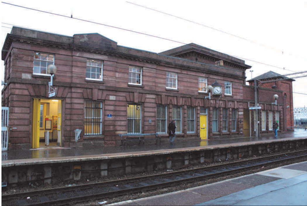
Figure 11: Edge Hill station (1836), north side buildings.
