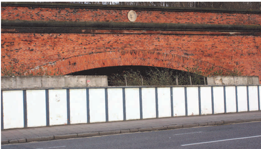
Figure 16: Railway bridge built by the L & YR to span the Waterloo tunnel (1849), Great Howard Street.
