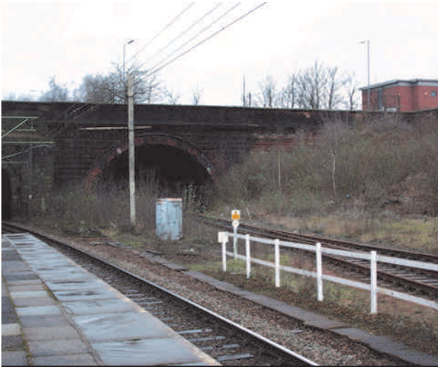
Figure 7: The Victoria tunnel portal on the right with one to Lime Street on the left, Edge Hill Station.
