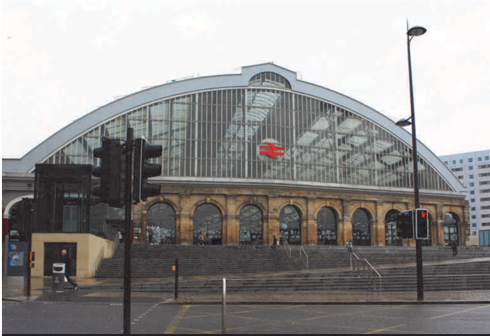
Figure 13: Entrance to Lime Street Station.
