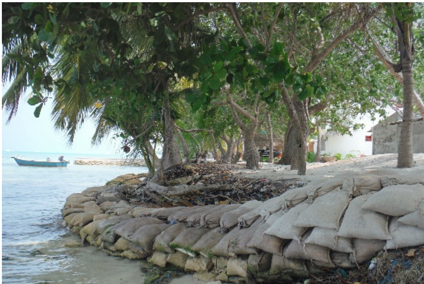
Photo 3 Installation of sandbags on the coastline
